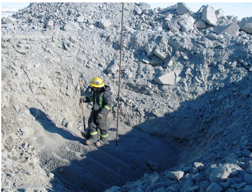
Photo 6: Setting base ND-SMP-160-DS. Frozen core material visible behind worker
