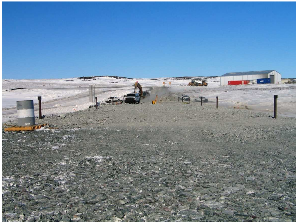
Photo 1: North dam facing north. Excavator is installing the last survey monument.
